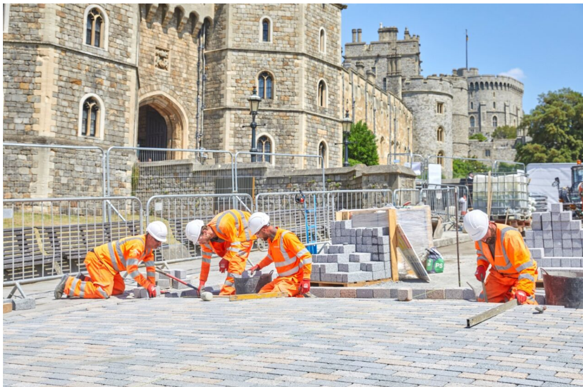
Improvement works at Castle Hill, Windsor
